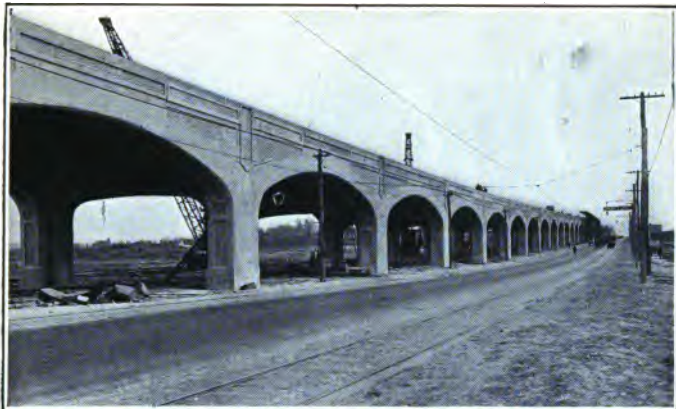
ELEVATED RAILROAD, CONCRETE MASONRY VIADUCT
